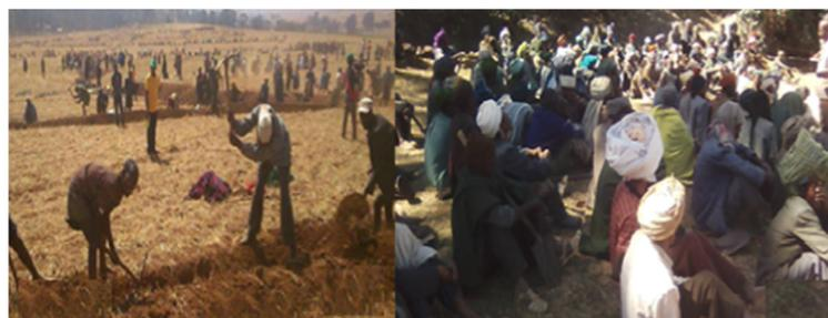
**Fig. 7** Community participation in watershed management in the Rib watershed. Construction of cut-off-drains for diversion of runoff coming from upstream areas and to trap sediments (left
